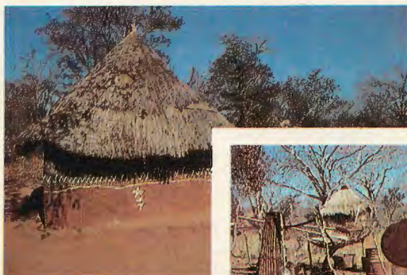
Typical African mud, wattle and thatch hut on Klipspringer Ranch, site of author's first job.
